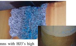
pour concrete to rebuild the columns, or (2) wrapping the columns with HJ3's high strength s-glass system. After attempting the traditional steel and concrete repair, the plant determined that the carbon fiber would be 75% to 80% less expensive.
