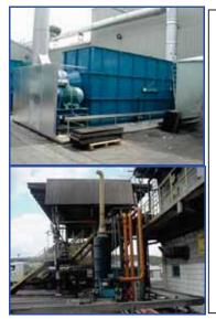
Design, supply and installation of complete filtration systems, comprising filter vessels fan, heat exchanger, chimney, all associated control system instrumentation.
