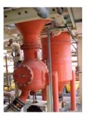
**Begg Cousland Venturi +** Cyclone system in U.K. removing HCI mist and TiO2 particulate.
