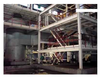
The Becoflex Discharge Vessel with single tangential inlet duct
