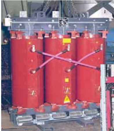
Cast Coil Transformer
