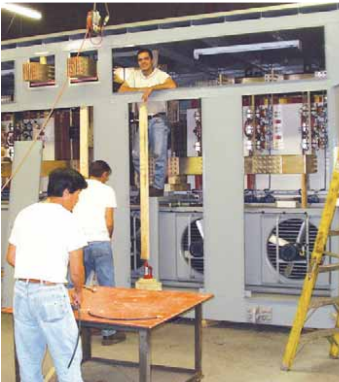
30 KA @ 233 VDC 12 pulse supply - Bleach Supply
